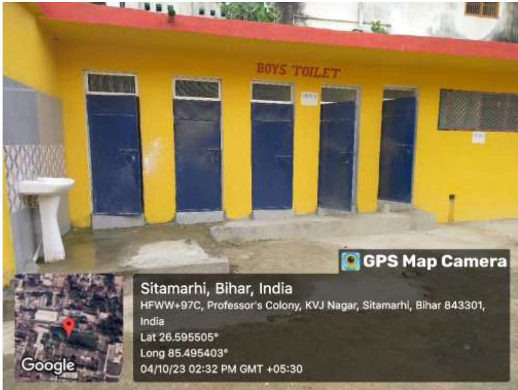
Fig 3B Disabled Friendly Barrier free clean and hygienic Boys Toilet
