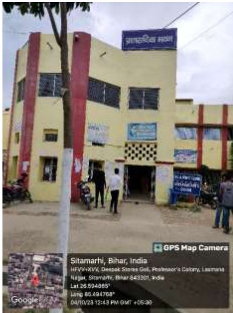
Fig 3 D Neat and Clean Administrative Building
