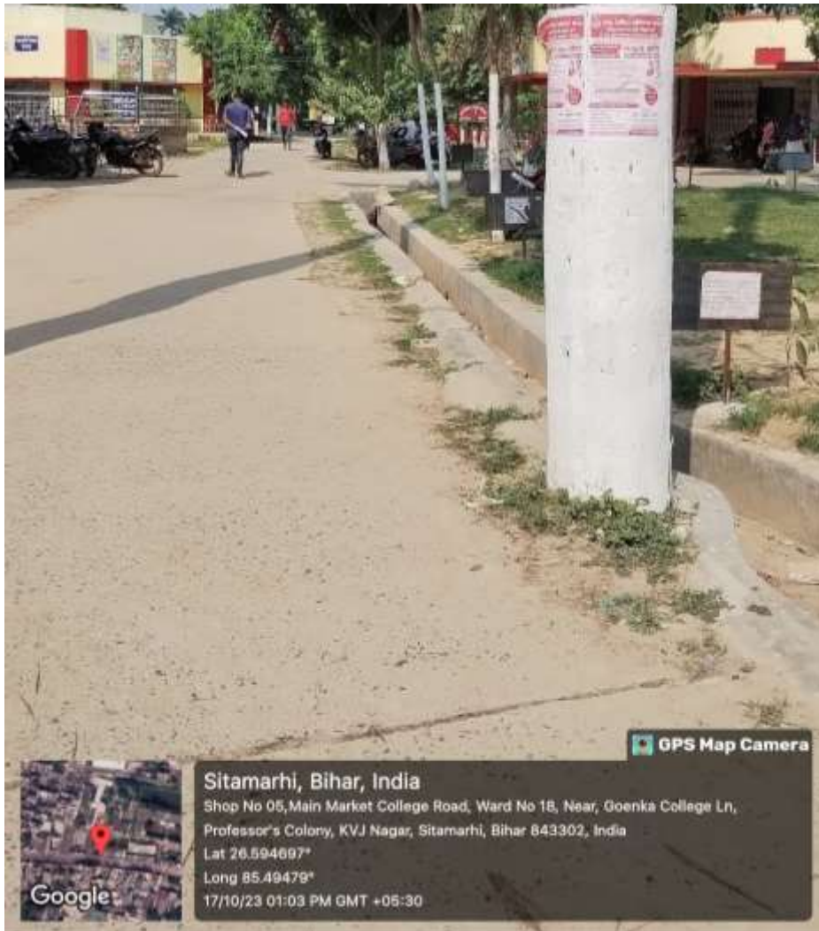
Fig 4 Rain Water Harvesting and channelling to water catchment area /pond neat clean green campus
